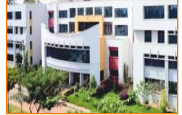
BMS Institute of Technology and Management (BMSIT&M) Avalahalli, Yelahanka Bangalore-560 064 Ph: +91 80 28561576
